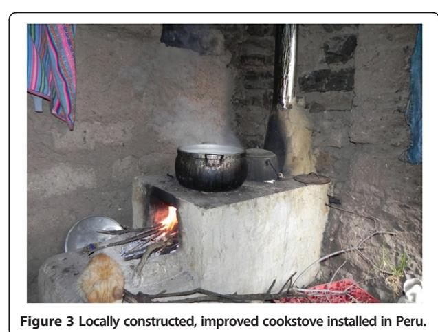
**Figure 3** Locally constructed, improved cookstove installed in Peru.
