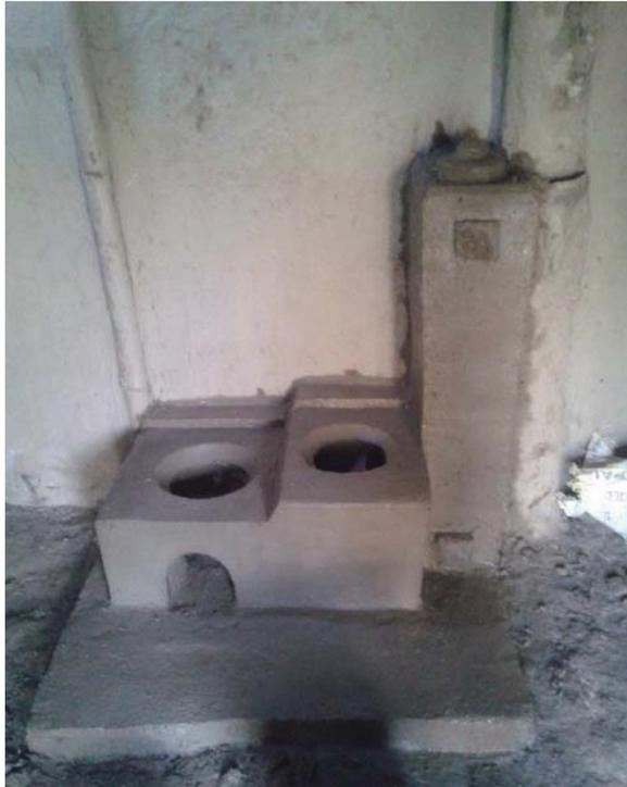
**Figure 4** Locally constructed, improved cookstove installed in Nepal.
